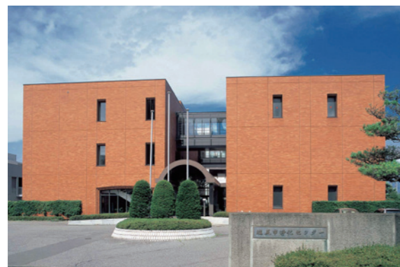
Shiojiri City Sewage Purification Center (Shiojiri City, Nagano Prefecture)
