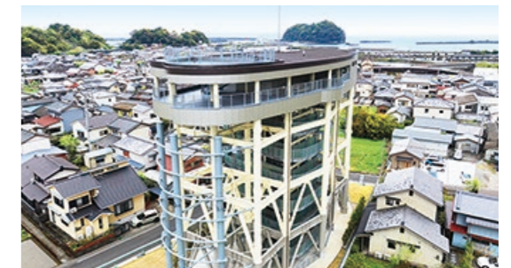
Kochi Prefecture, Tsunami Evacuation Tower
