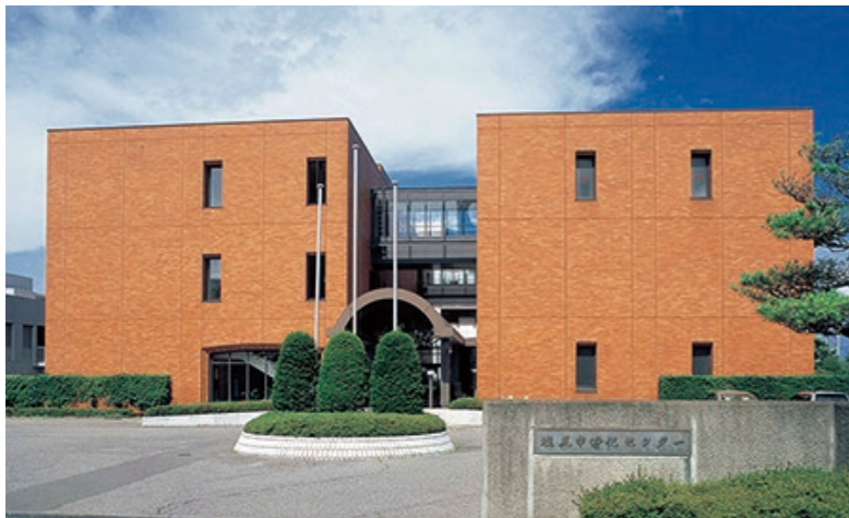
Sewage Purification Center (Shiojiri City, Nagano Prefecture)
