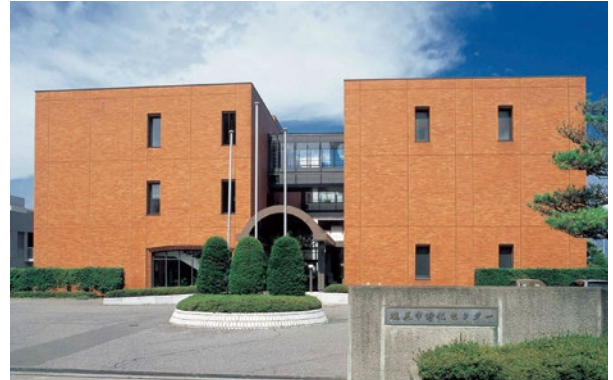
Sewage Purification Center (Shiojiri City, Nagano Prefecture)
