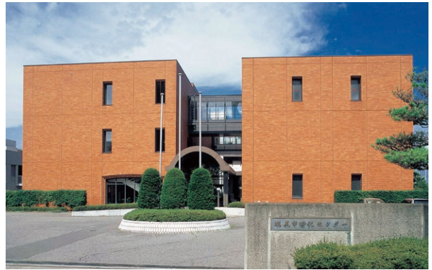
Sewerage Purification Center (Shiojiri City, Nagano Prefecture)
