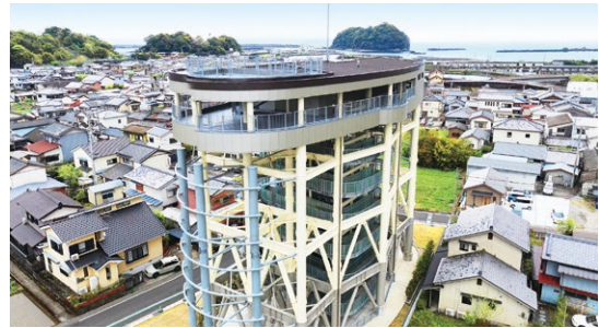
Kochi Prefecture, Kuroshio Town, Tsunami Evacuation Tower
