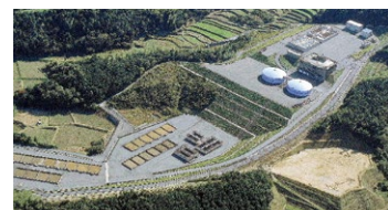
Hizumi Purification Plant (Yanai Water Supply Authority)
