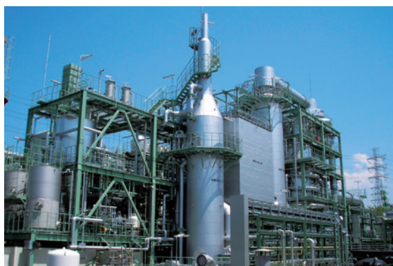
Sewage Sludge Gasification System in Kiyose Water Reclamation Center (Tokyo)
